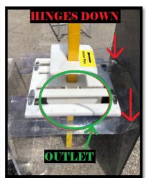
Once the unit is removed and the sediment is cleaned out, you can reinstall the unit. Clean off the grates of debris and ensure the grate slots are perpendicular to the lowest outlet pipe.
